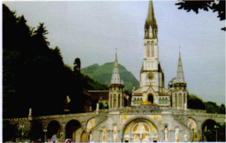
The 25,000 capacity underground St. Pius X Basilica
